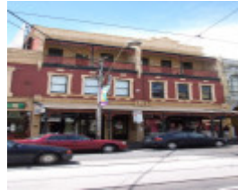
Bridge Rd 37-43 853.JPG
