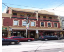
Bridge Rd 37-43 853.JPG
