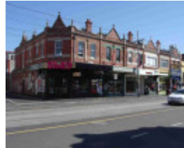
Fitzroy Brunswick Street 377- 387.JPG
