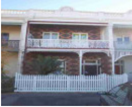
fitzroy north bennett street fitzroy north bennett street 51
