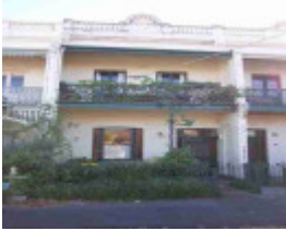
fitzroy north bennett street fitzroy north bennett street 55
