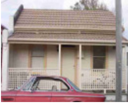
fitzroy north eastham street fitzroy north eastham street 12
