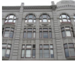
Elaborate detailing on the eastern face
