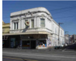
Fitzroy Brunswick Street 393.JPG
