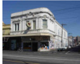
Fitzroy Brunswick Street 393.JPG
