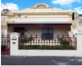
fitzroy north liverpool street fitzroy north liverpool street 26
