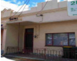
fitzroy north liverpool street fitzroy north liverpool street 27
