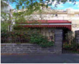
fitzroy north liverpool street fitzroy north liverpool street 28
