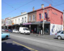
Fitzroy Brunswick Street 305- 319.JPG
