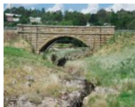
NEWTOWN BRIDGE PRECINCT SOHE 2008
