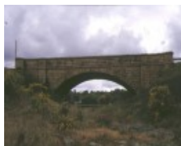
newtown bridge precinct beechworth side elevation
