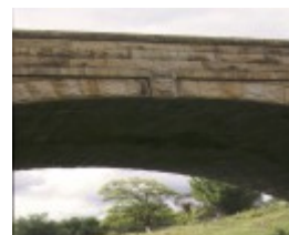
newtown bridge precinct beechworth detail of bridge arch & keystone
