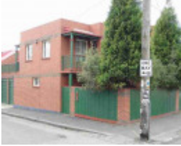
fitzroy kerr street fitzroy kerr street 127-129
