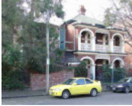
fitzroy moor street fitzroy moor street 45 unit 1
