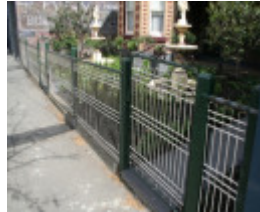
Fence - 513 Brunswick Street
