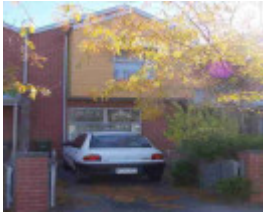
fitzroy north bennett street fitzroy north bennett street 97
