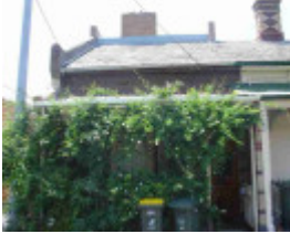
fitzroy north bennett street fitzroy north bennett street 100
