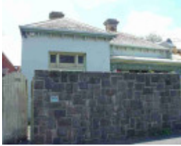
fitzroy north bennett street fitzroy north bennett street 104
