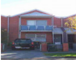
fitzroy north bennett street fitzroy north bennett street 105
