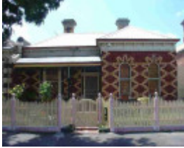
fitzroy north bennett street fitzroy north bennett street 106
