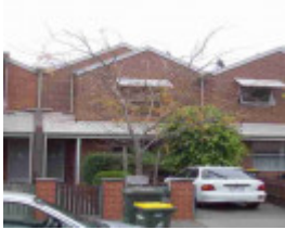
fitzroy north bennett street fitzroy north bennett street 107
