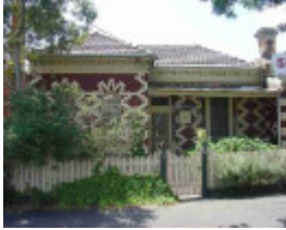
fitzroy north bennett street fitzroy north bennett street 108
