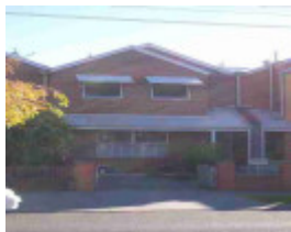
fitzroy north bennett street fitzroy north bennett street 109
