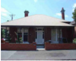
fitzroy north bennett street fitzroy north bennett street 110
