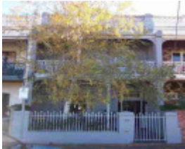
fitzroy north bennett street fitzroy north bennett street 59
