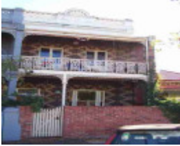
fitzroy north bennett street fitzroy north bennett street 61
