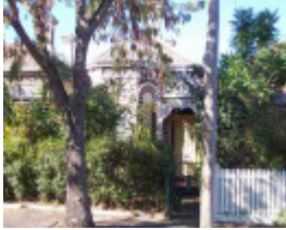
fitzroy north bennett street fitzroy north bennett street 62
