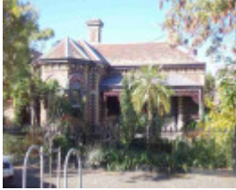
fitzroy north bennett street fitzroy north bennett street 64
