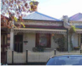
fitzroy north bennett street fitzroy north bennett street 65
