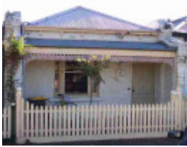
fitzroy north bennett street fitzroy north bennett street 67
