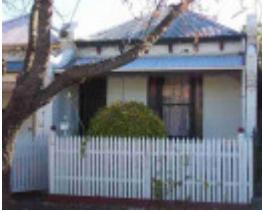
fitzroy north bennett street fitzroy north bennett street 69
