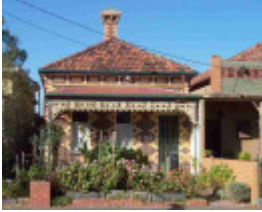
fitzroy north bennett street fitzroy north bennett street 70
