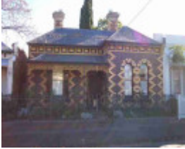
fitzroy north bennett street fitzroy north bennett street 71
