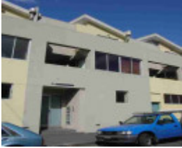
fitzroy fitzroy street fitzroy fitzroy street 494 unit 1
