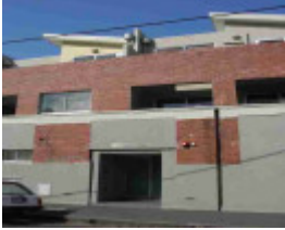
fitzroy fitzroy street fitzroy fitzroy street 496 unit 1
