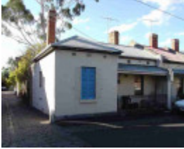
fitzroy garfield street fitzroy garfield street 1
