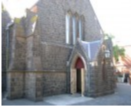
ST STEPHENS ANGLICAN CHURCH SOHE 2008
