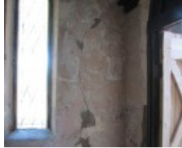
ST STEPHENS ANGLICAN CHURCH SOHE 2008
