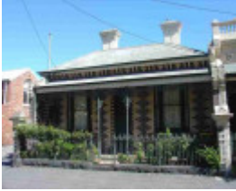
carlton north newry street carlton north newry street 67
