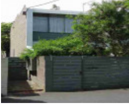
richmond richmond terrace richmond richmond terrace 79 unit 1
