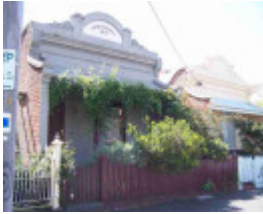
carlton north ogrady street carlton north ogrady street 28
