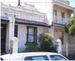
carlton north ogrady street carlton north ogrady street 32
