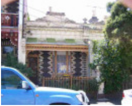
carlton north ogrady street carlton north ogrady street 44
