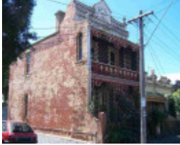
carlton north ogrady street carlton north ogrady street 46
