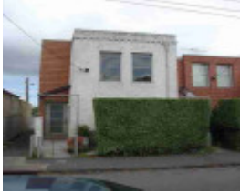
richmond the crofts richmond the crofts 12a
