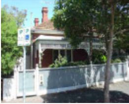
carlton north park street carlton north park street 474
