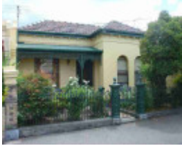
carlton north station street carlton north station street 655
