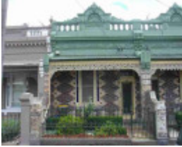
carlton north station street carlton north station street 523
