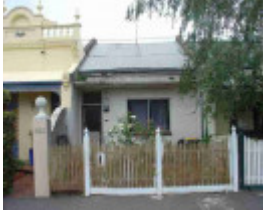
carlton north station street carlton north station street 348
