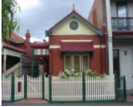
carlton north station street carlton north station street 670
