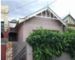
carlton north station street carlton north station street 678
